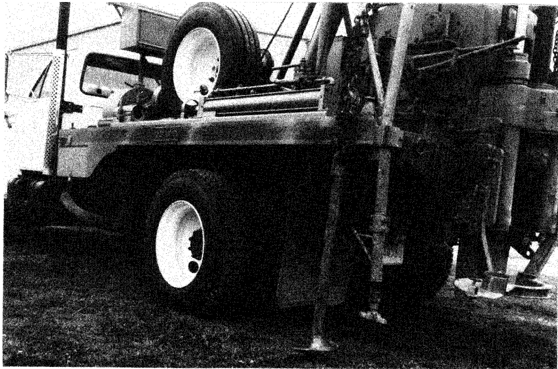
Figure 6-2. Photograph of screw-type earth anchors fastened to the drill rig with load binders to anchor the rig
